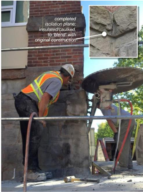
Figure 8. Sawcutting equipment with inset showing final joint at the isolation plane
